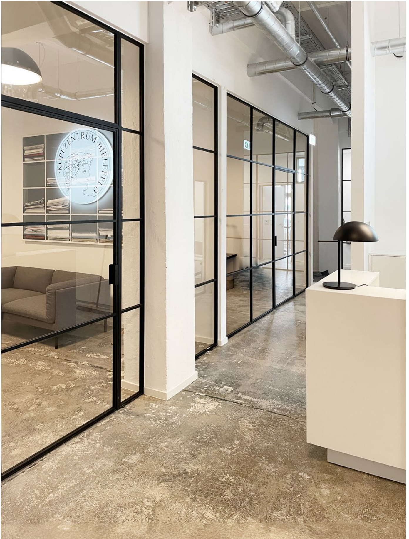
▲ Hinged door 1-leaf + fixed elements + skylights Timeless 2 mullion, clear glass | SLIM frame | black, RAL 9005, matt, fine texture | SLIM handle, 160 mm
